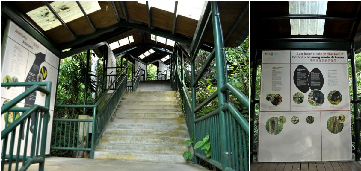
Left: Newly replaced roof at the staircase. Right: Translucent roofing to allow natural lighting for signage along the staircase.
