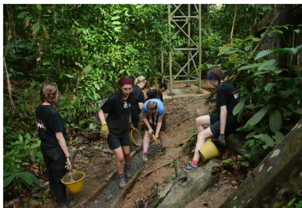
BATs volunteers repairing the perimeter walkways around the forest enclosure.
