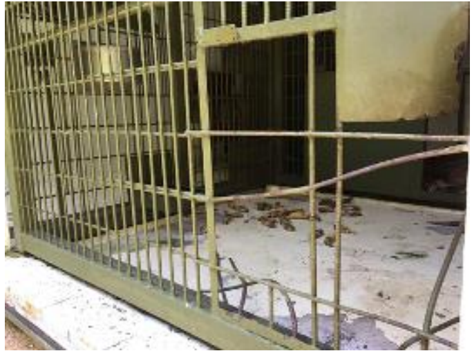
Cage bars destroyed and bent by translocated bear Abai at quarantine cage-9, BSBCC.
