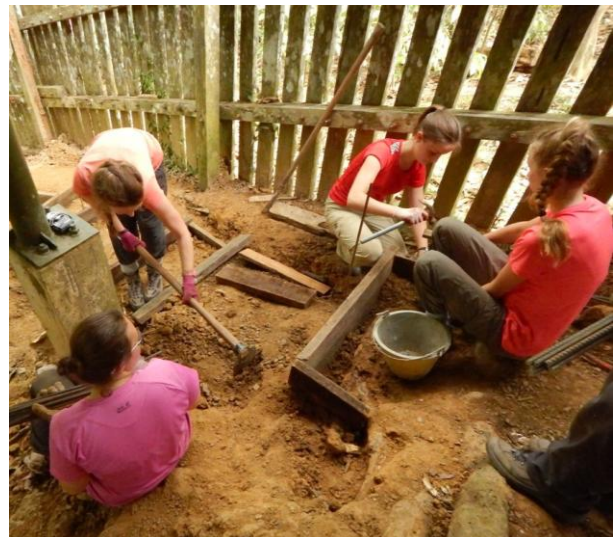
BATs volunteers building steps outside the forest enclosure.
