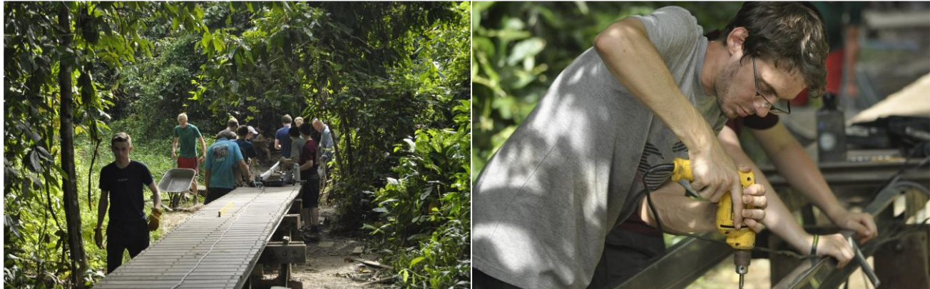
Left: BATs volunteers constructing the perimeter boardwalk for the proposed new forest enclosure. Right: Architect intern from Arkitrek, Jonathan Dolan assisting in the construction of the perimeter boardwalk.
