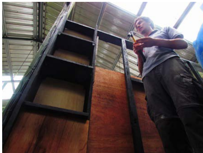
Volunteer Ronan building the cabinet at the new bear house.
