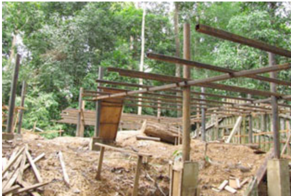
Footings and frame for the observation platform under construction during November 2011.
