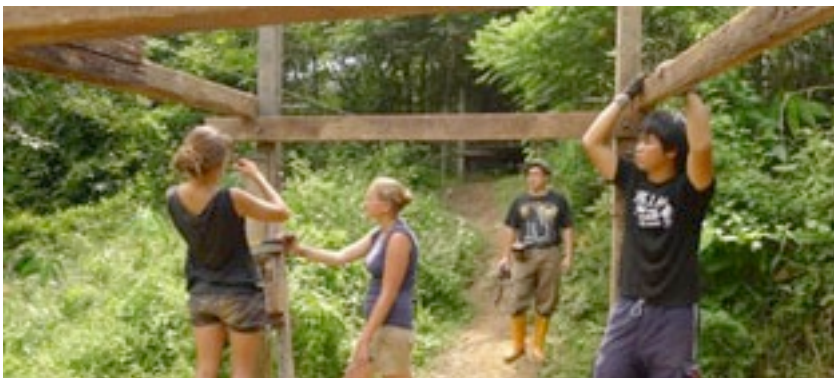
Raleigh volunteers working on post construction under the access boardwalk.
