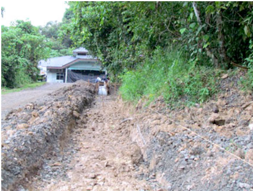
Roadside drainage work in progress.
